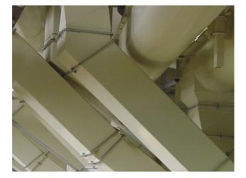
FM Square pipes are supplied from 160 x 160 mm to 400 x 400 mm in the following lengths: 470 mm, 970 mm and 1470 mm.
